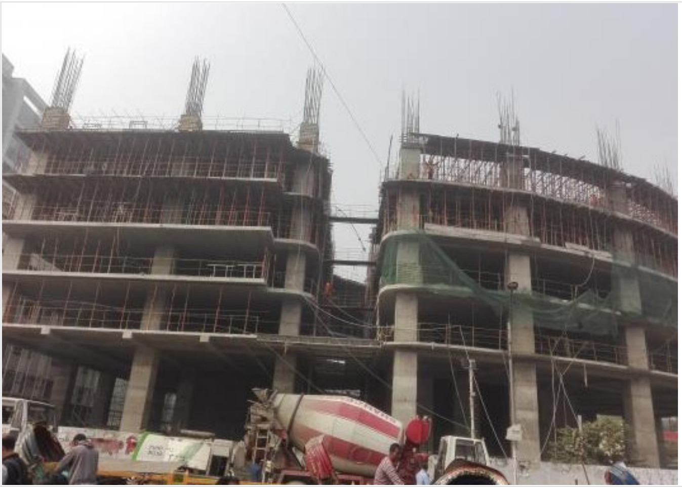
Project Picture on 24-01-21
