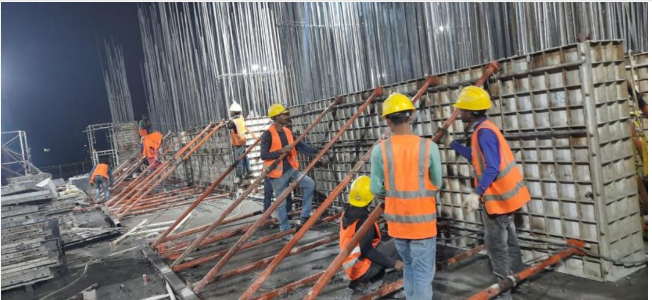
Lift Core Wall Shuttering on 17-01-21
