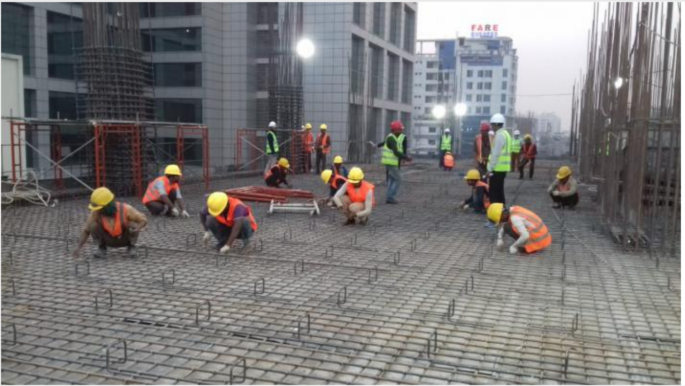
Slab Re-bar Work on 30-01-21
