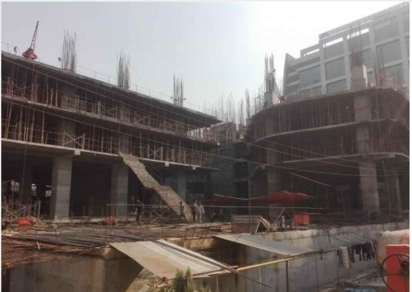
3rd Floor South Tower Stair Complete on 11-01-21
