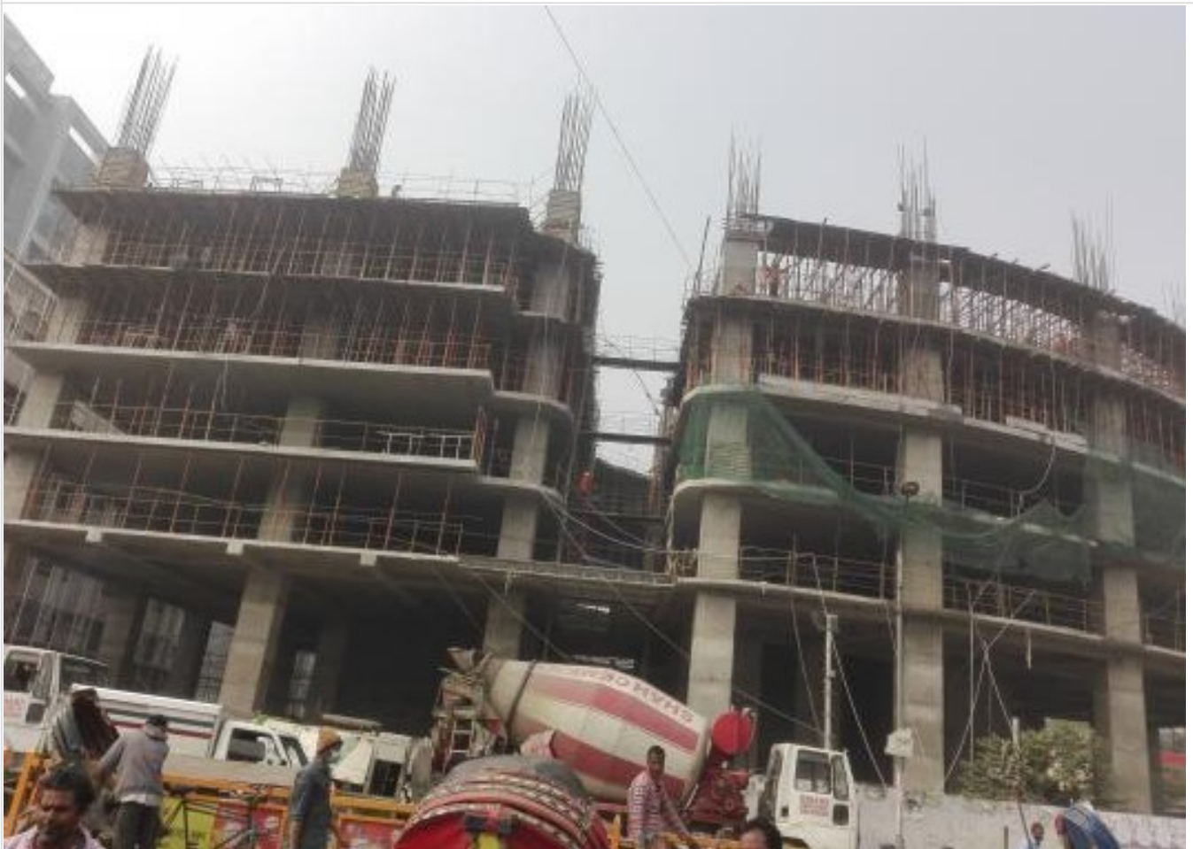
Project Picture on 24-01-21
