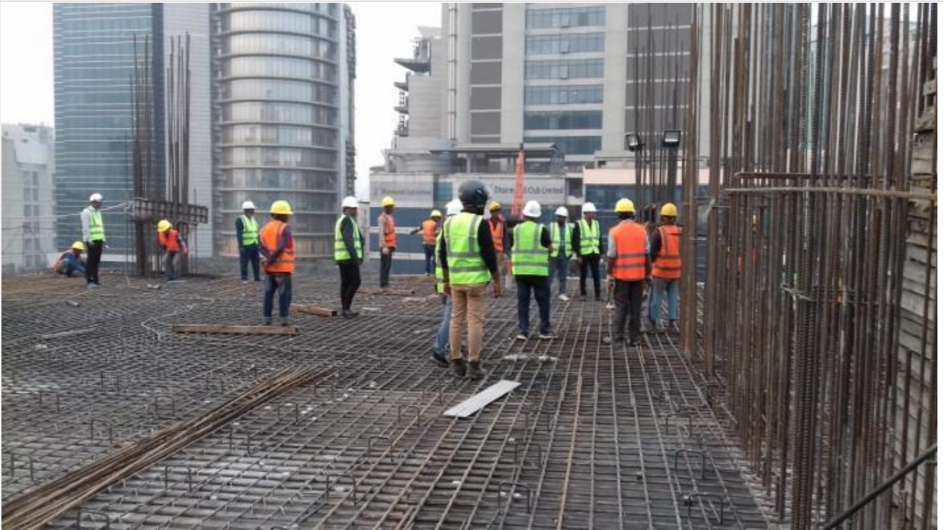
Work Inspection on 30-01-21
