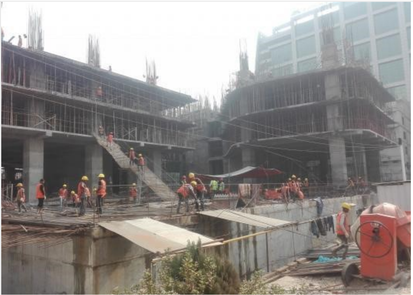
Project View from West Side on 06-02-21
