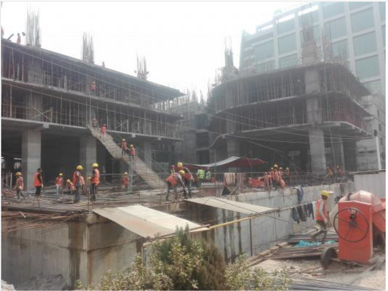
3rd Floor South Tower Lift Core Complete on 06-01-21
