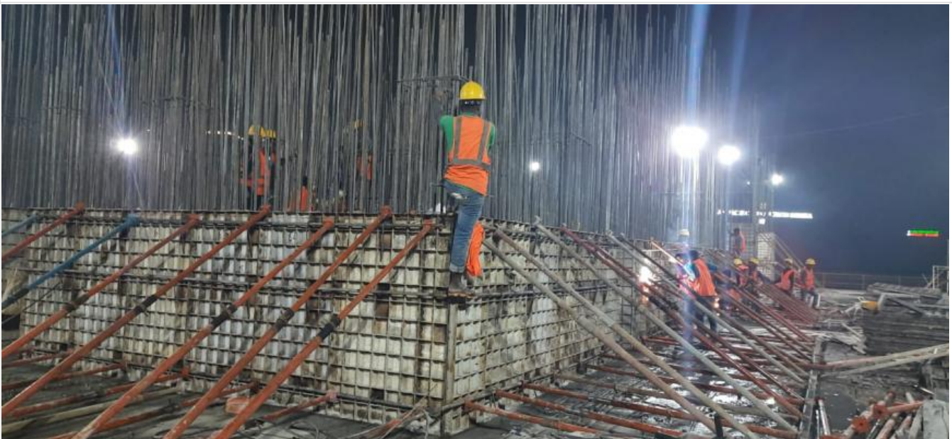
Lift Core Wall Shuttering on 16-01-21
