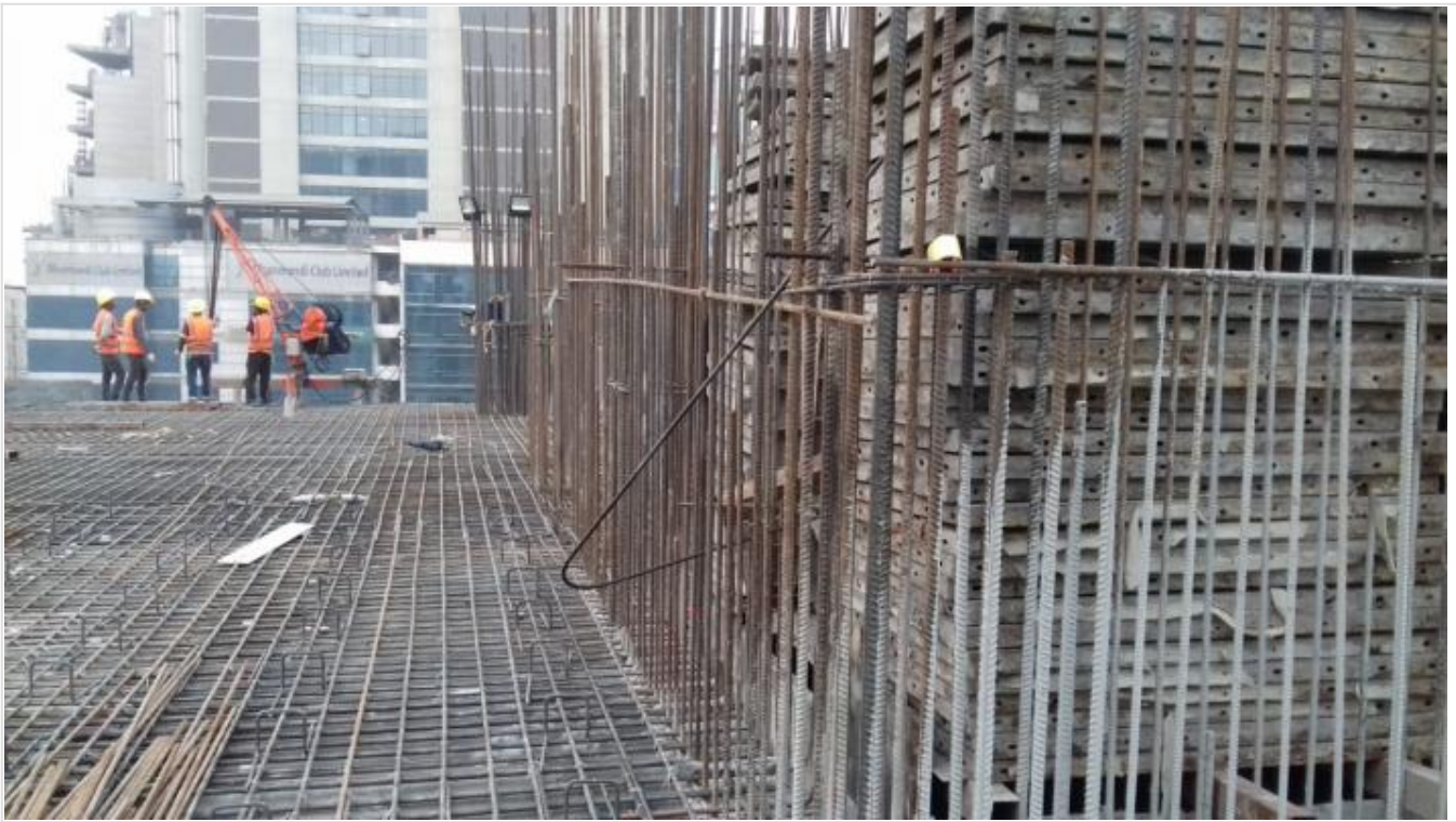
Roof Slab on 01-02-21
