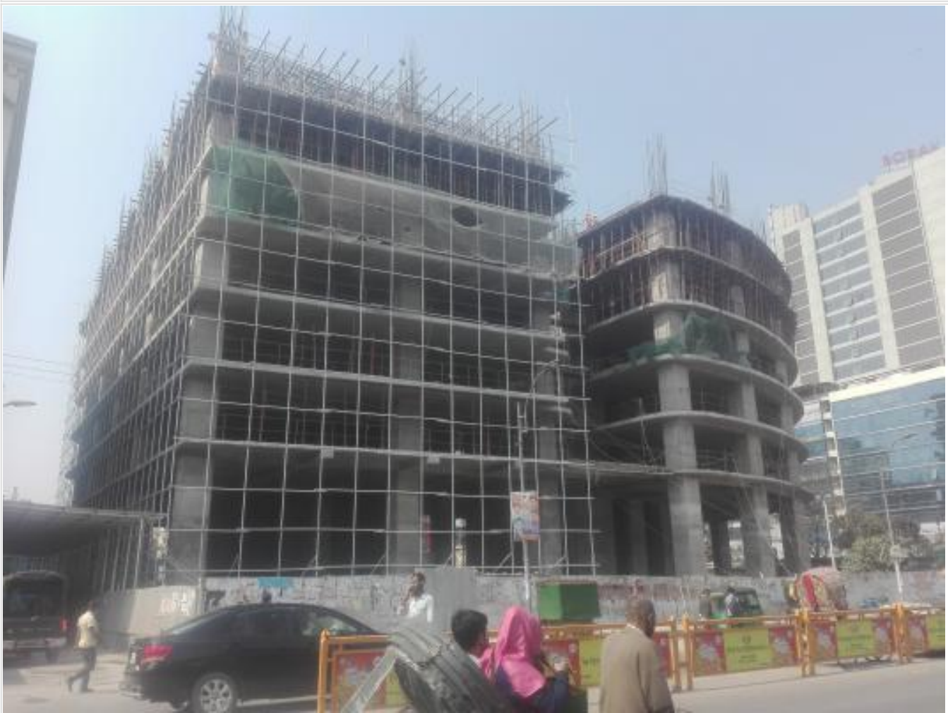
Project View from East Side on 06-02-21
