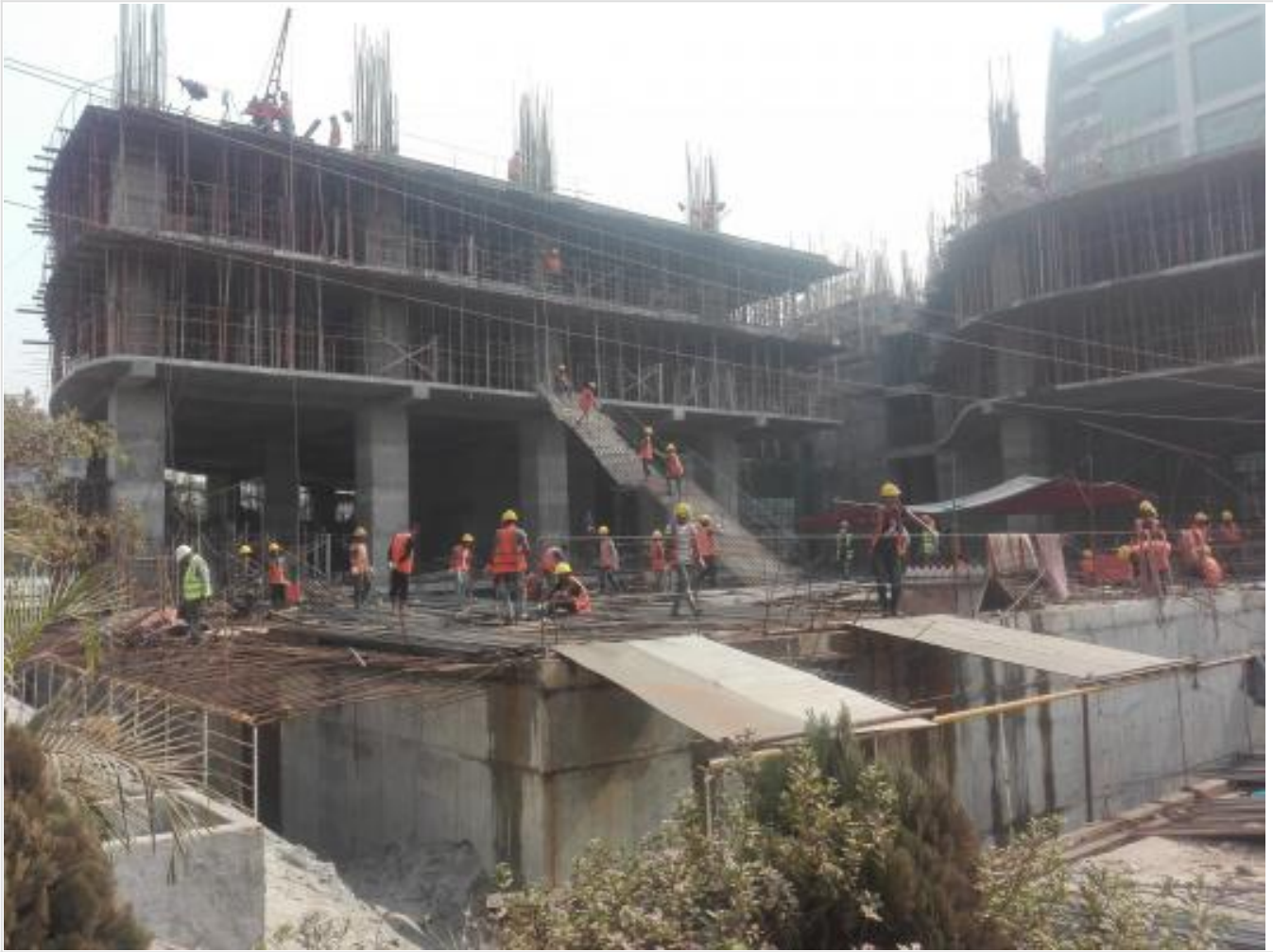
3rd Floor South Tower-Column Complete on 06-01-21
