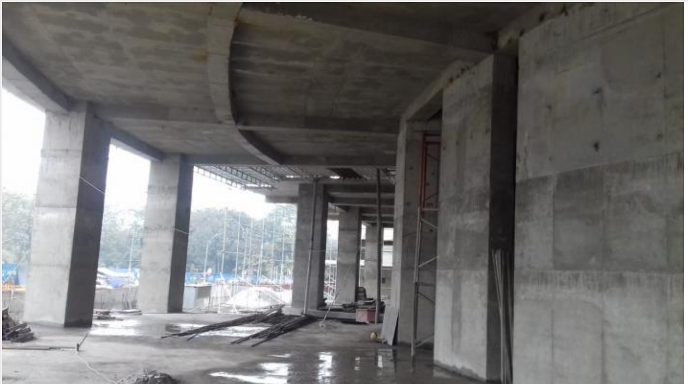
Inside Building on 29-01-21
