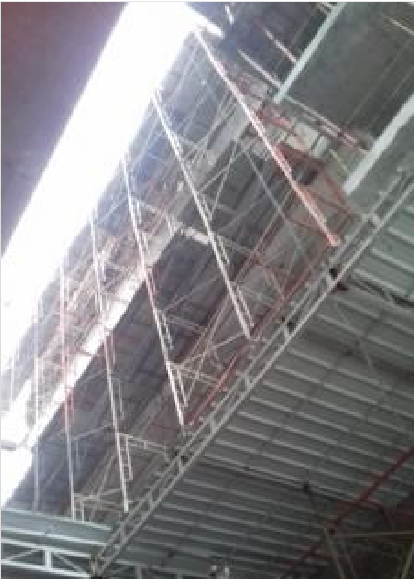
Safety Railing on 03-02-21
