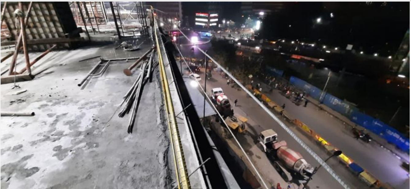
Night Shift Working on 16-01-21
