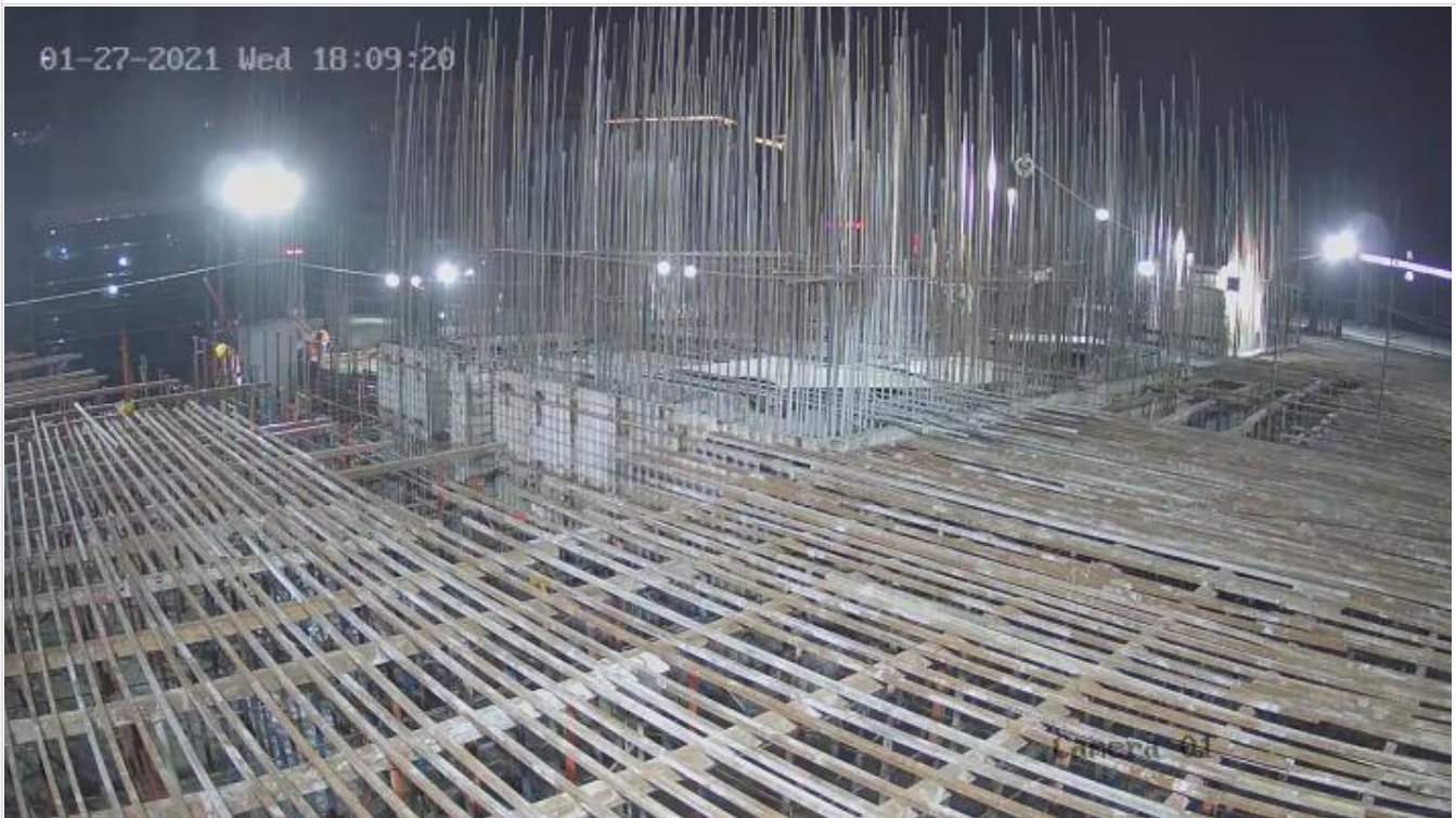
Slab Shuttering on 27-01-21
