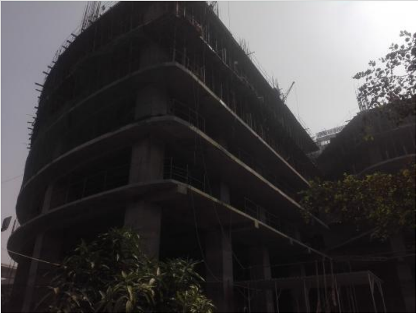
Project Picture on 03-02-21
