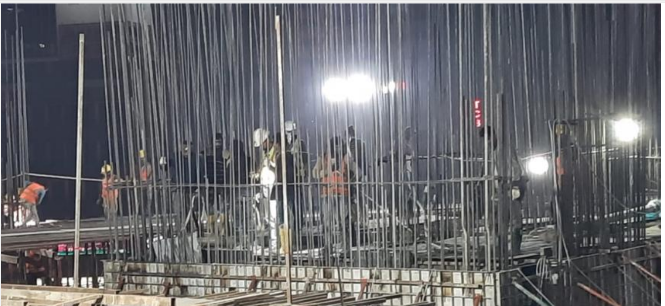
Re-bar Work on 18-01-21
