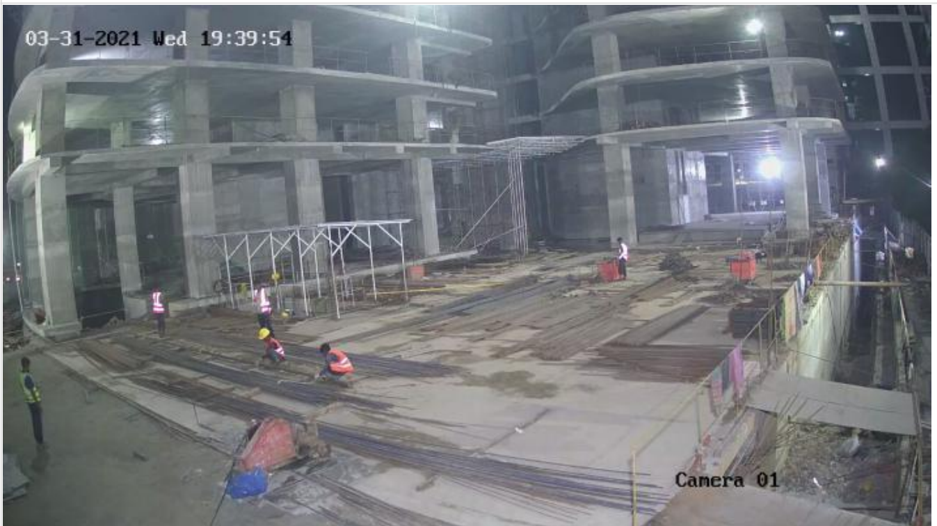
Night Shift Working on 31-03-21
