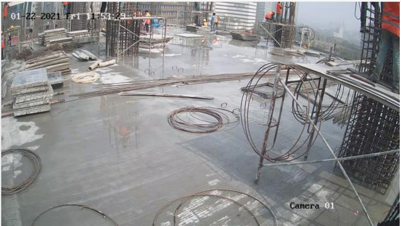
Curing after 4F South Tower Slab Concret on 22-01-21
