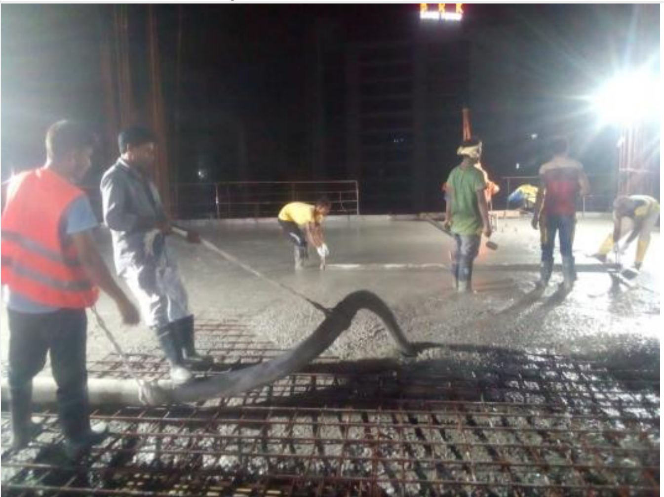
South Tower 11th Floor Slab Concreting on 02-09-21
