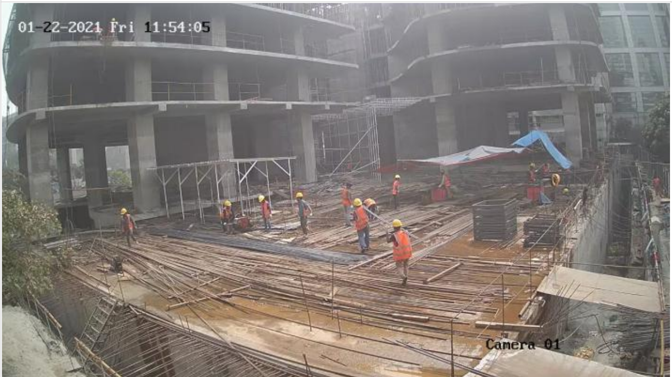
Re-bar Work on 22-01-21
