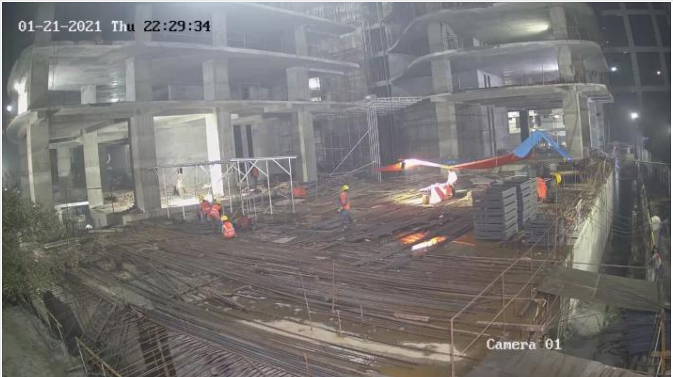
Night Shift Working on 21-01-21
