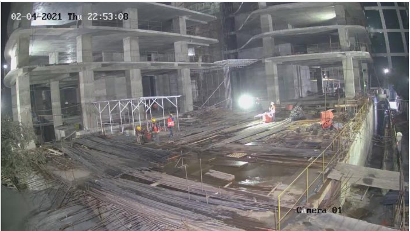
Night Shift Working on 04-02-21
