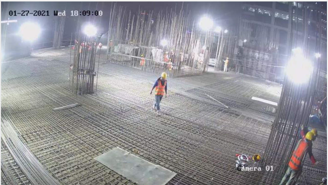
Slab Re-bar Work on 27-01-21
