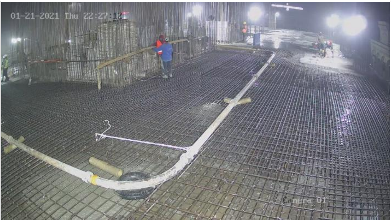
South Tower 4th Floor Roof Slab Concreti on 21-01-21
