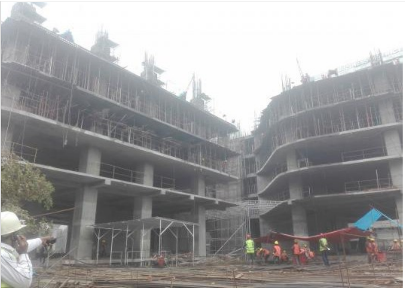
South Tower 4th Floor Roof Slab Running on 20-01-21
