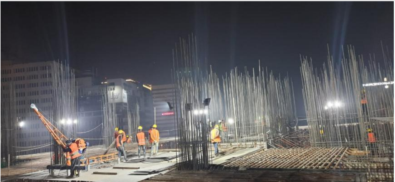
Re-bar Lifting by Roof Hoist on 14-01-21
