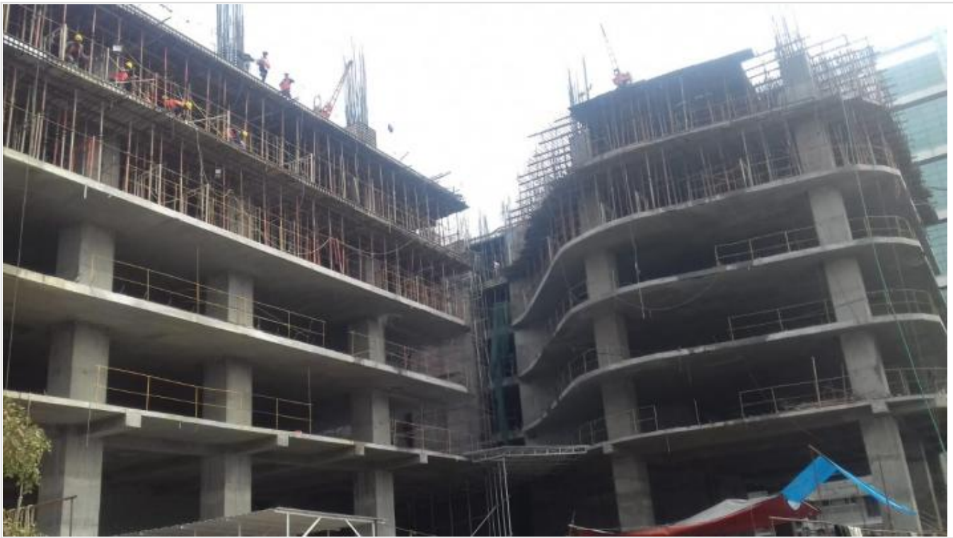
Project Picture on 29-01-21
