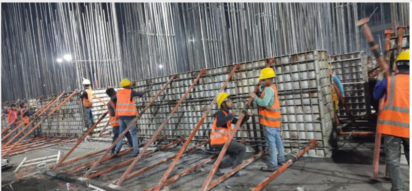
Lift Core Wall Shoring on 14-01-21
