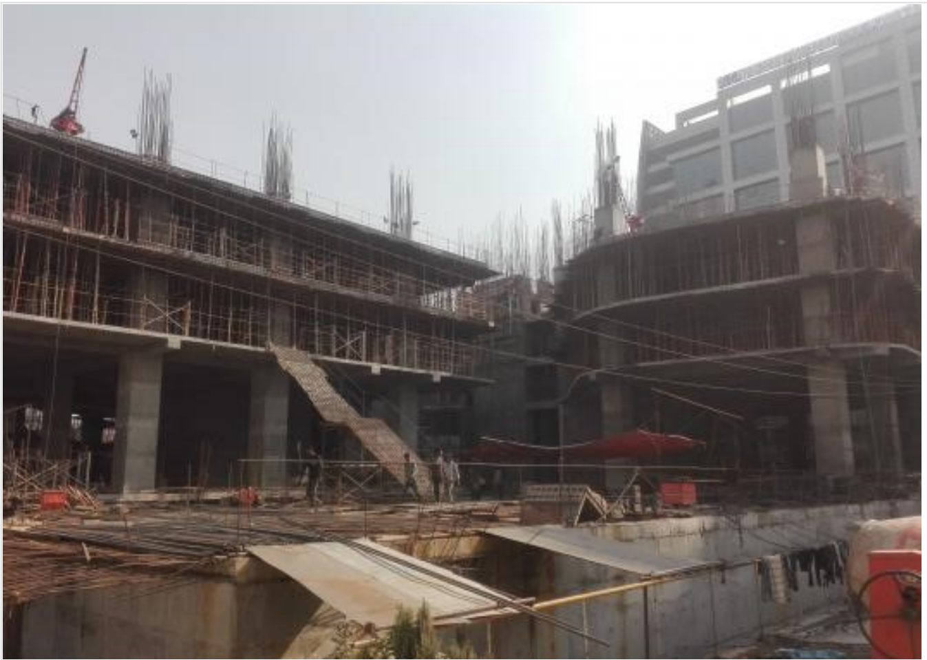
3rd Floor South Tower Slab Complete on 11-01-21
