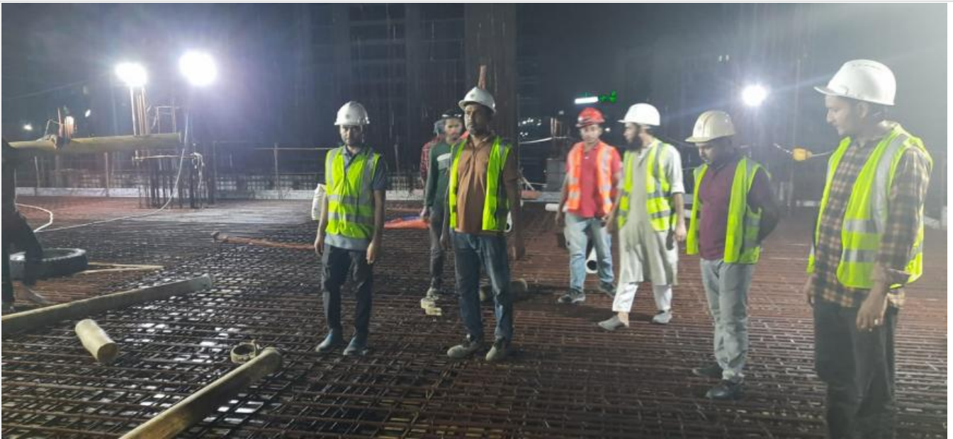
South Tower 11th Floor Slab Concreting on 02-09-21
